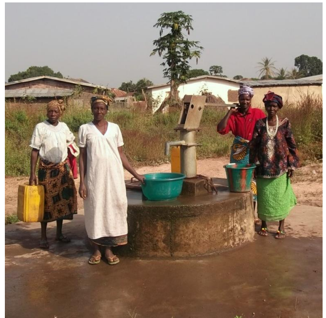
NEW WATER WELL CONSTRUCTED BY SDGO IN SINKUNIA
